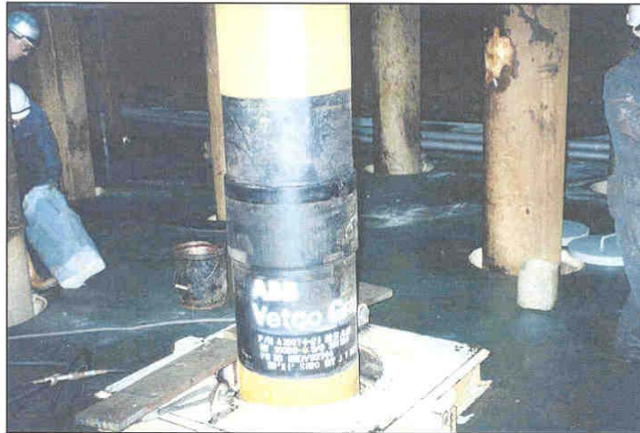
Vetco SR20 connector at work station awaiting installation of low profile SL type wrap.
