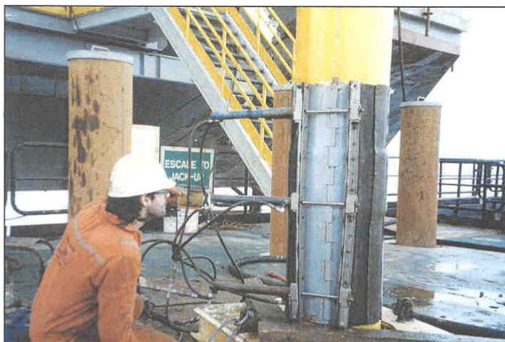
Locking bar in position. Technician releasing pressure from hydraulic jacks.
