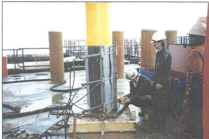
Low profile wrap positioned loosely over SR20 connector. Note the gap between each end of wrap.
