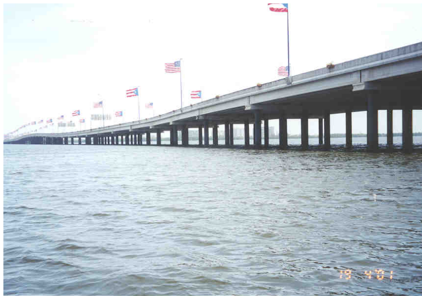
Moscoso Bridge 1.6 miles dual expressway (405) 42" piles
