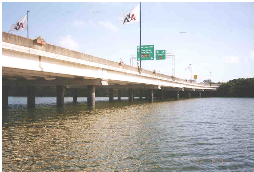
Moscoso Bridge with wraps installed Aeropuerto/San Jose end showing Isle Verde mangroves.
