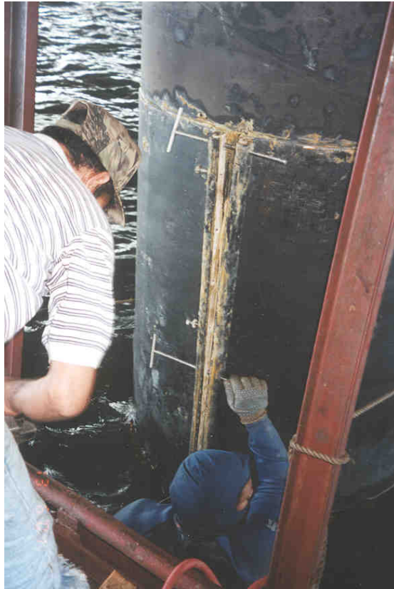
Diver removing line up rod prior to driving lag fasteners
