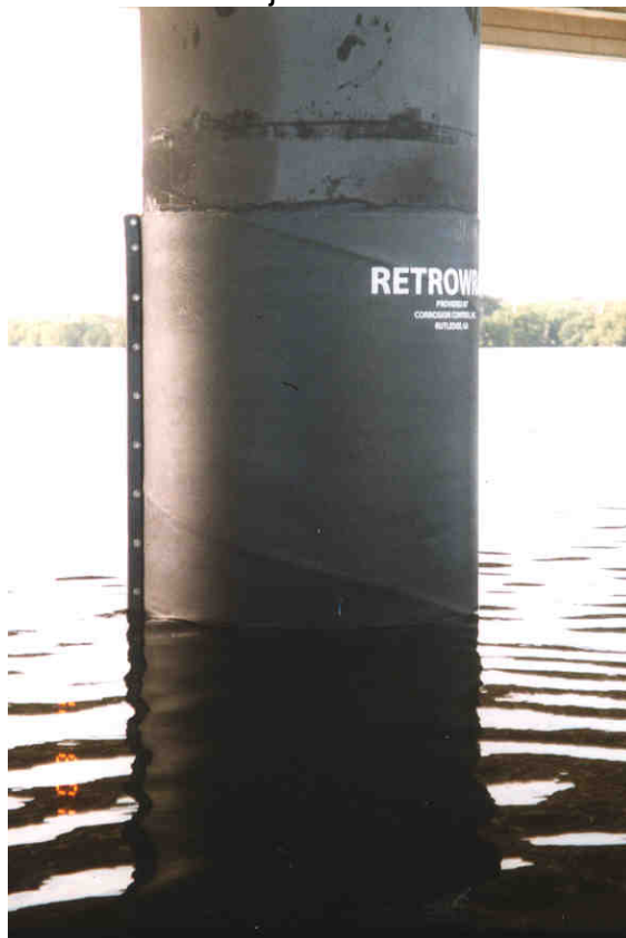
Installed Retrowrap showing closure flange with fasteners fully installed. Also shown is product name and client identification information.
