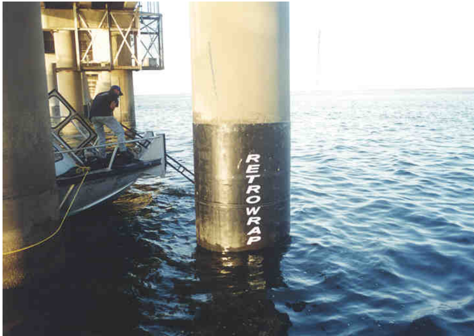
Before and After! Note Outline of Pile Joint Clearly Visible
