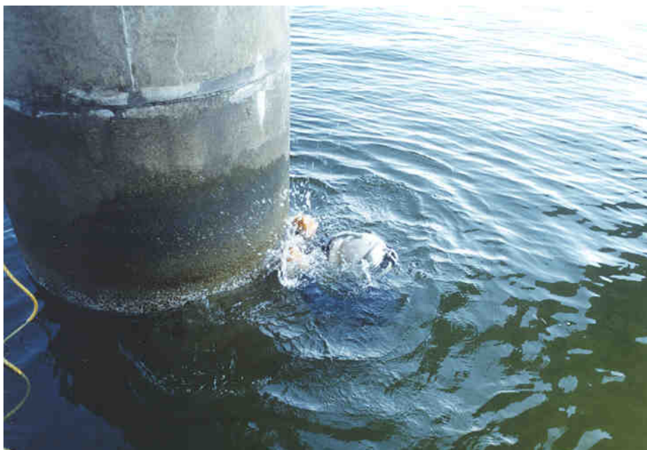
Diver hand scraping marine growth from pile. LP water jet would be the recommended production procedure.
