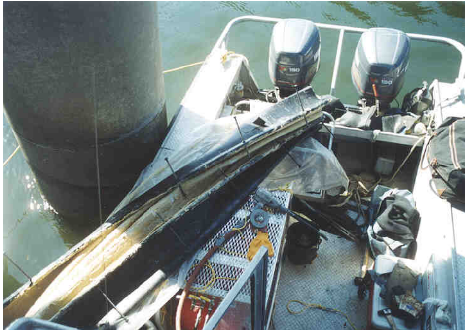
The 54"Ø x 10 (141 ft. 2 ) Retrowrap showing hydrophobic thixotropic gel impregnated inner layer and removable draw bolts preinstalled in opposing closure flanges.
