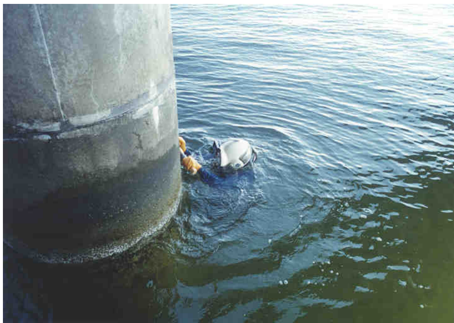
Diver hand scraping marine growth from pile. LP water jet would be the recommended production procedure.
