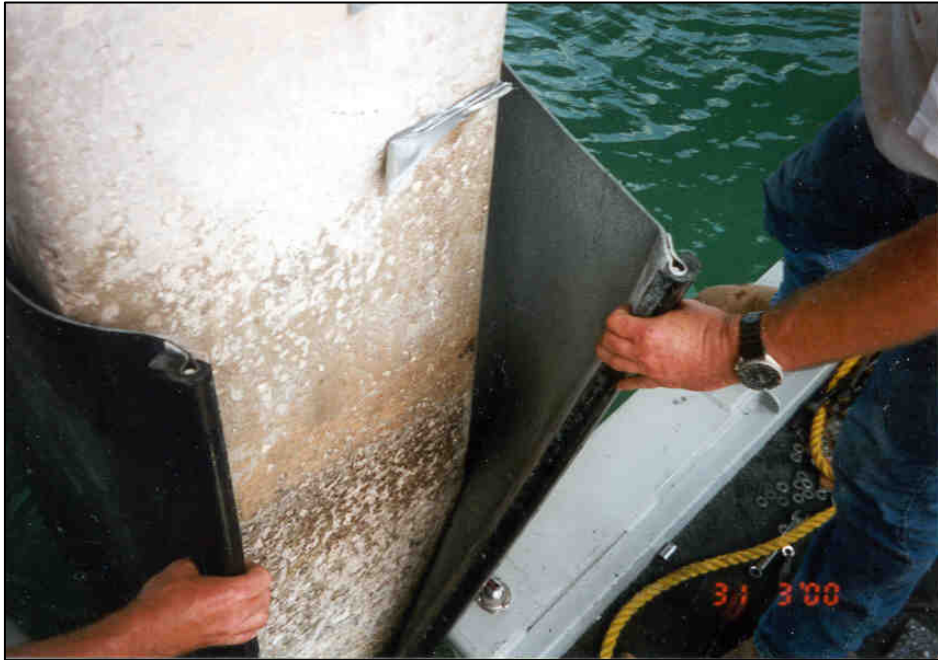
Anode wrap with zinc lined inner face clearly visible being positioned around pile.
