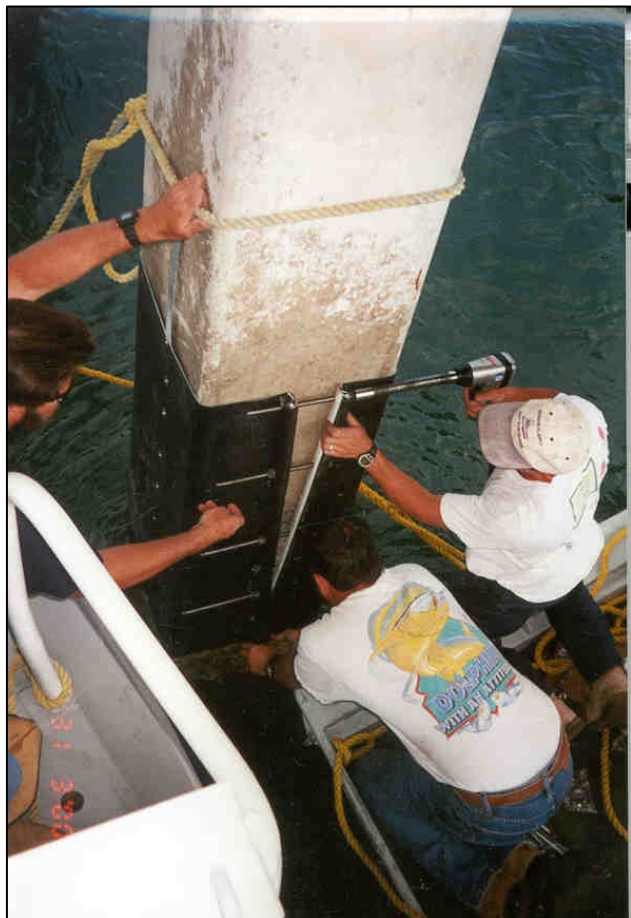
Anode wrap with zinc lined inner face clearly visible being positioned around pile.
