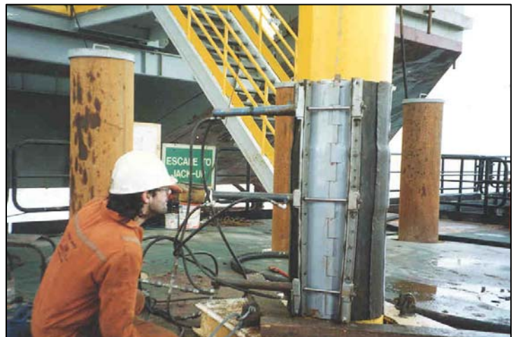
Locking bar in position. Technician releasing pressure from hydraulic jacks.
