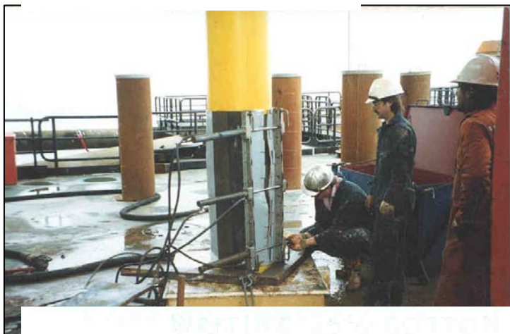
Low profile wrap positioned loosely over SR20 connector. Note the gap between each end of wrap.
