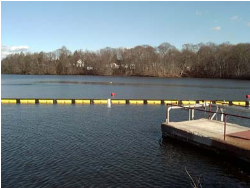
Heavy Duty Debris Barrier installed at Lake Whitney, Hamden CT to help protect their intake screens.
