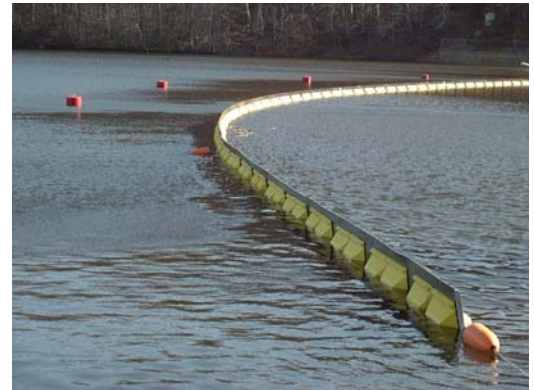
Heavy Duty Debris Barrier installed at Lake Whitney, Hamden CT to help protect their intake screens.
