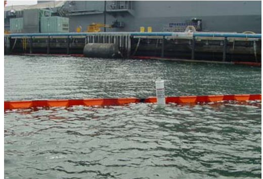
The new Force Protection Boom installed in a highly sensitive area at US Navy San Diego Submarine Base .
