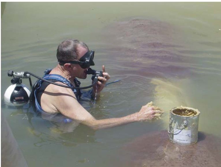
Application of hydrophobic Retrogel P to pipe joint weight coat before installation of adjustable end seals.
